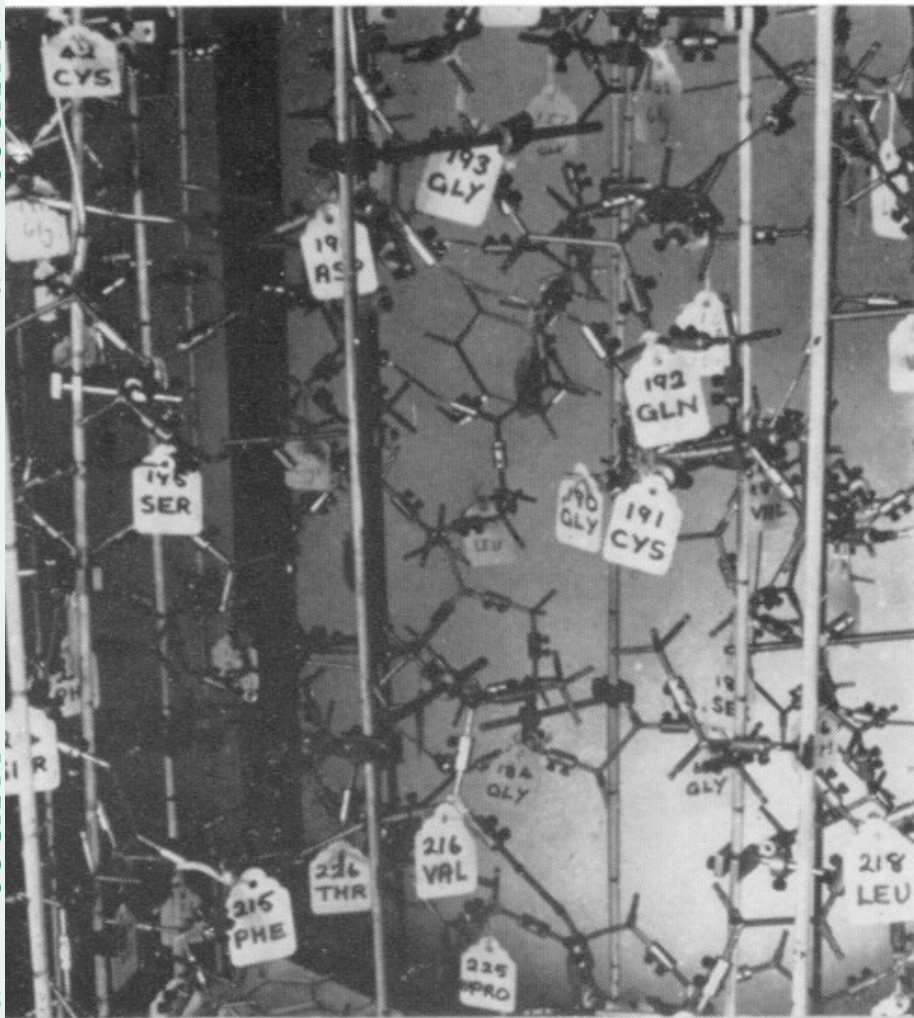
FIGURE 7. The 'tosyl-hole' of the hypothetical model of elastase. Note that Val-216 (replacing Gly-216 in chymotrypsin) blocks the entrance to this hole.
